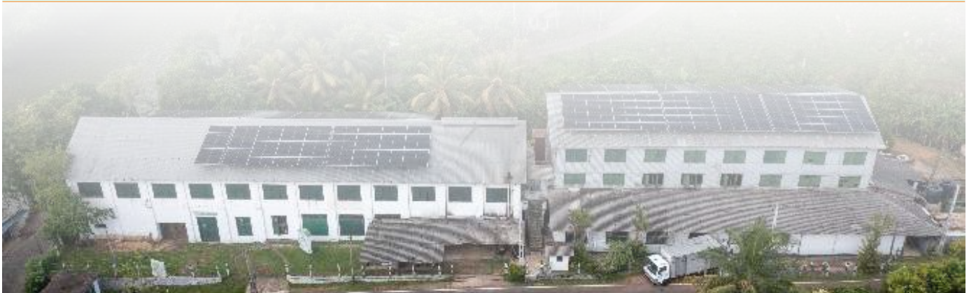
Neuchatel Rubber Processing Center Rooftop Solar System
