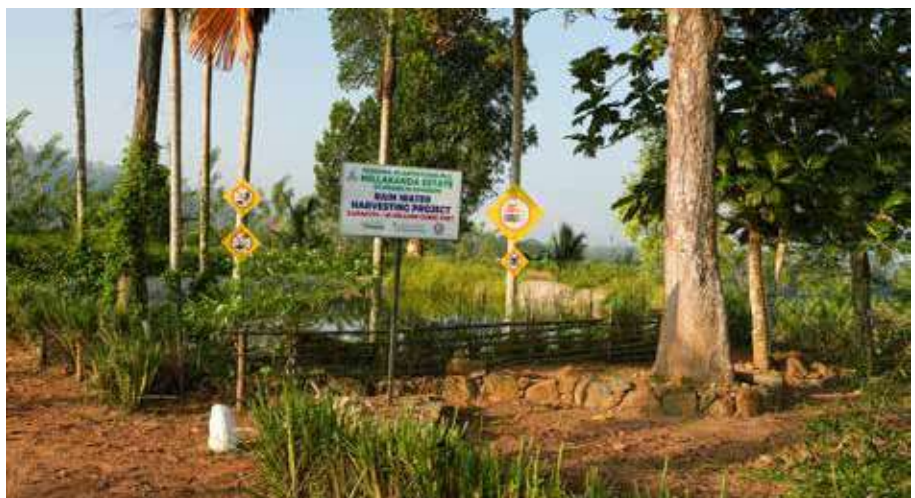
Rainwater Harvesting Pond
